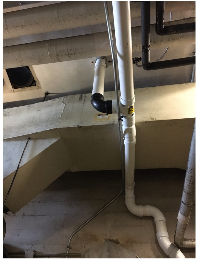
Vent pipe routing in the Boiler room to the fan location on the roof.
