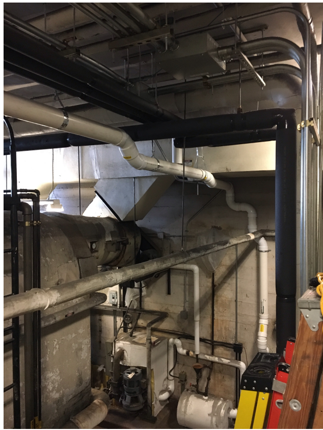
Vent pipe routing in the Boiler room to the fan location on the roof.
